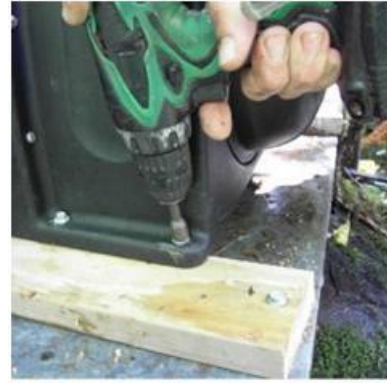
Fixing a turbine to a timber base
