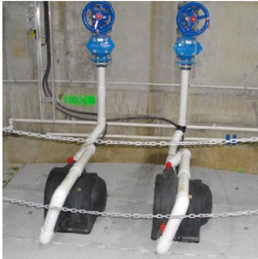
Dual install, one unit runs on 30m (98 ft) head the other 10m (33 ft) head
