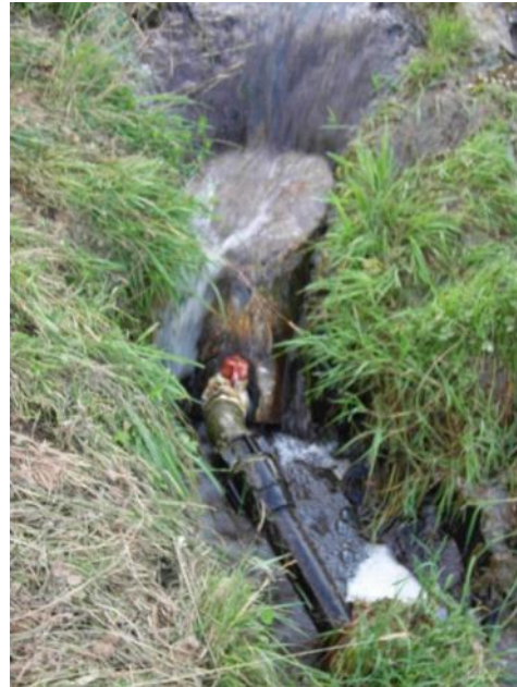
Intake made from stainless steel scrap
