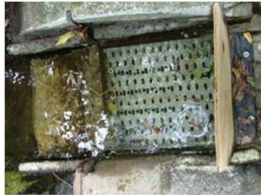
Perforated galvanized cable tray intake
